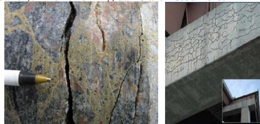
Figure 1- some samples of cracking because of stones Alkali reaction.
